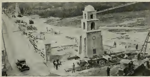
General View of Bridge. Old Bridge Between Lines of Temporary Barriers and Far Railing
